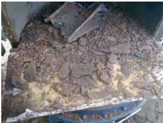
Collapsed fire damper
