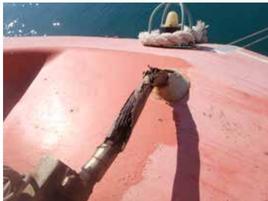
Lifeboat cable protective cover corroded
