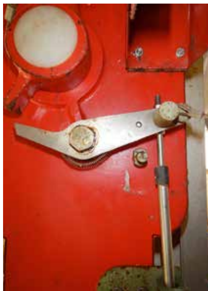
Lifeboat hydrostatic on-load release mechanism locked in open-maintenance position
