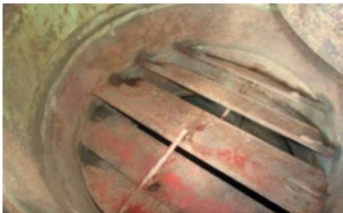
Fire Safety is the deficiency category with the most detainable deficiencies found on DNV GL vessels in 2014 and fire dampers are the most frequent of these.
