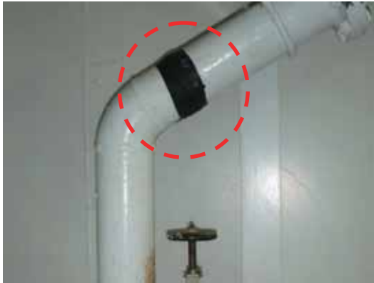
Pipe temporarily repaired with rubber patch
