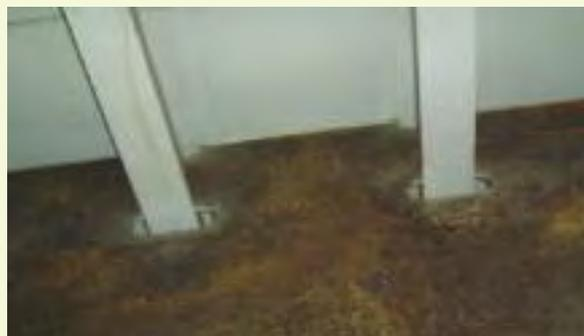
On closer inspection, however, the rust was found to be a surface layer of corroded steel grit. Light abrasion removed the rust to reveal a sound coating underneath.
