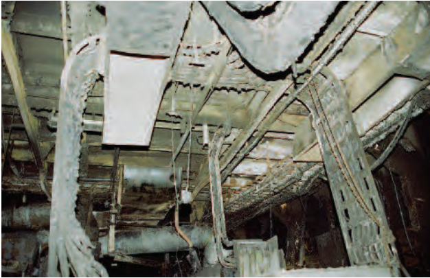
Fire spread along cable trays away from an auxiliary generator where the fire originated
