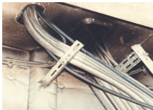
Cables entering a distribution board through fire stopped openings in the casing
