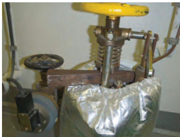
Quick closing valve held open with a steel wedge
