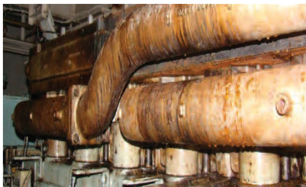
Exhausts completely uninsulated
