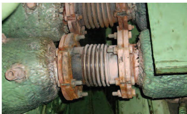
Exhaust bellows exposed
