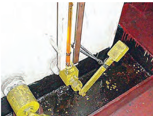
Self-closing gauge glass held open with string
