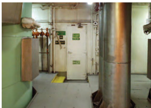
Poorly marked escape route and door
