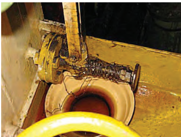
Self-closing gauge glass valve gagged with wire
