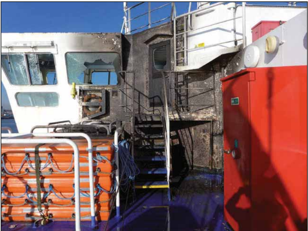
Figure 1: Damage caused by the fire
