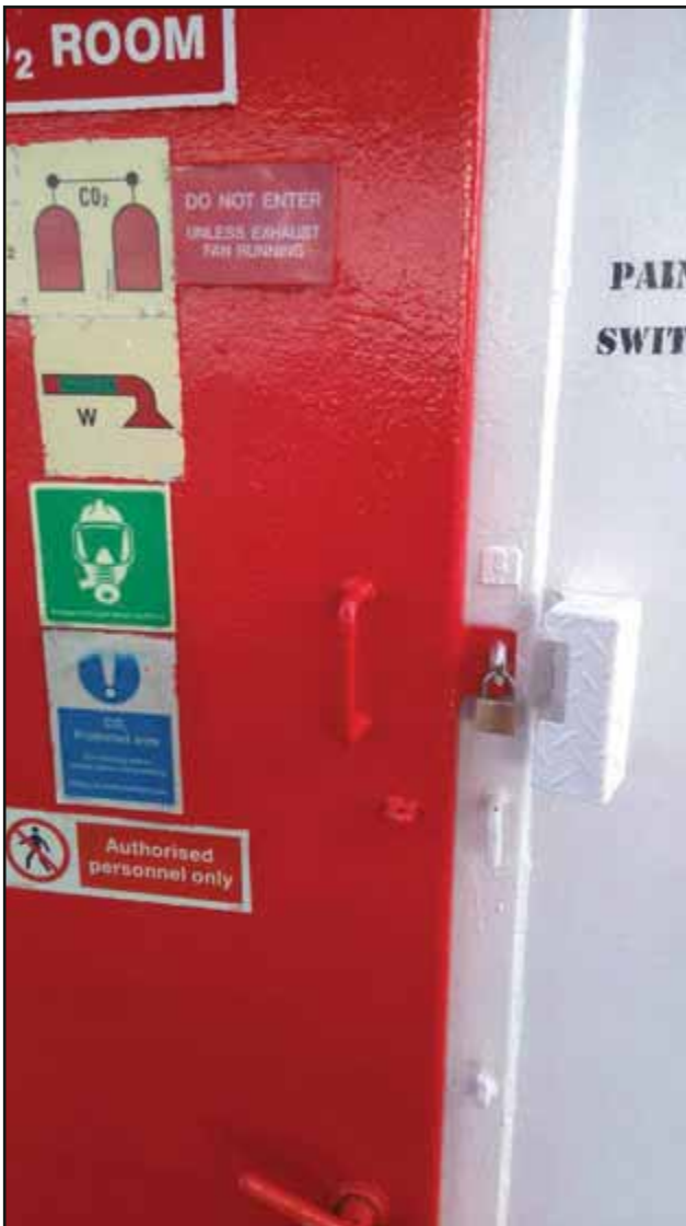
Figure 2: Access to CO 2 space
