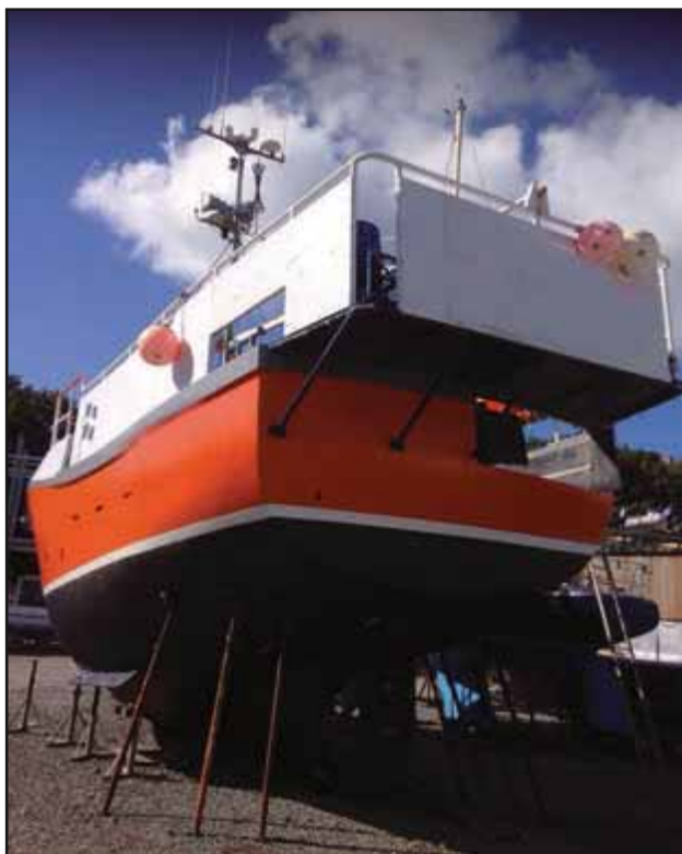
Figure 1: Opening in transom
