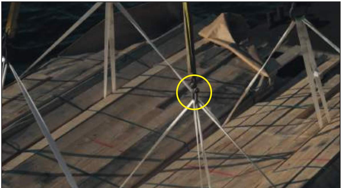
Figure 6: Open shackles used as cargo hooks
