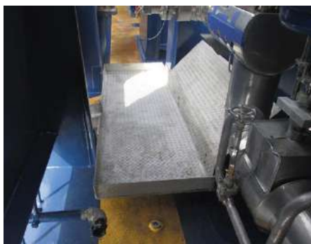
Figure 2.53 and 2.54 – Drip-trays – protection against cryogenic related hazards that may represent risk of local girder structural failure.
