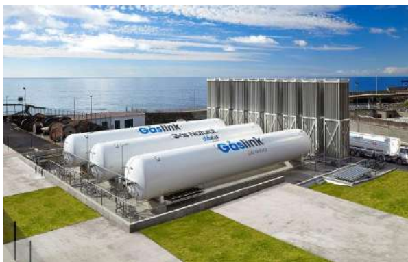
Figure 8.5 – Type-C tanks in small scale LNG installation (with visible evaporators) – for NG supply to the grid and LNG trucks (source: Grupo Sousa Gáslink)
