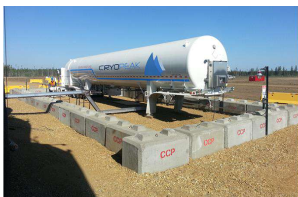
Figure 12.8 – LNG trainler semi-fixed installation. Despite not being a purely TTS bunkering operation it gives evidence on how flexible LNG trucks and trailer can be. Here a semi-fixed installation that may be used for LNG bunkering or fuelling. Typically an installation for LNG consumption more than bunkering/transfer.
