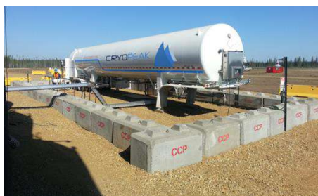
Figure 2.37, 2.38 and 2.39 – Two on the top representing fixed LNG bunkering installations, both with 3 horizontal pressure tanks. The one below representing an LNG trailer installed temporarily, with concrete defences and
