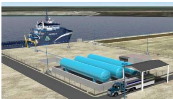
Figure 8.6 – Type-C tanks in fixed LNG bunkering installation. (source: Harvey Gulf)
