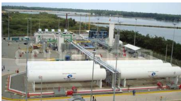
Figure 8.4 – Fixed LNG small scale installation, for LNG bunkering and grid supply – equipped with re-liquefaction plant.
