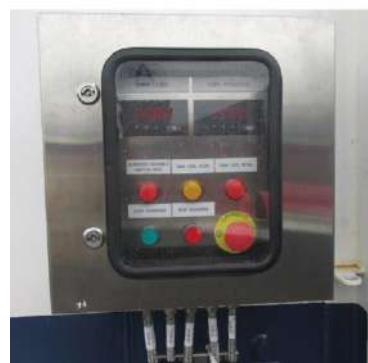
Figure 2.47 – ESD local command switchboard and alarm indicator [26]
