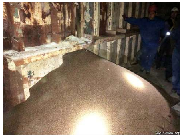
Candidate photo for Deficiency Photo of the Year
