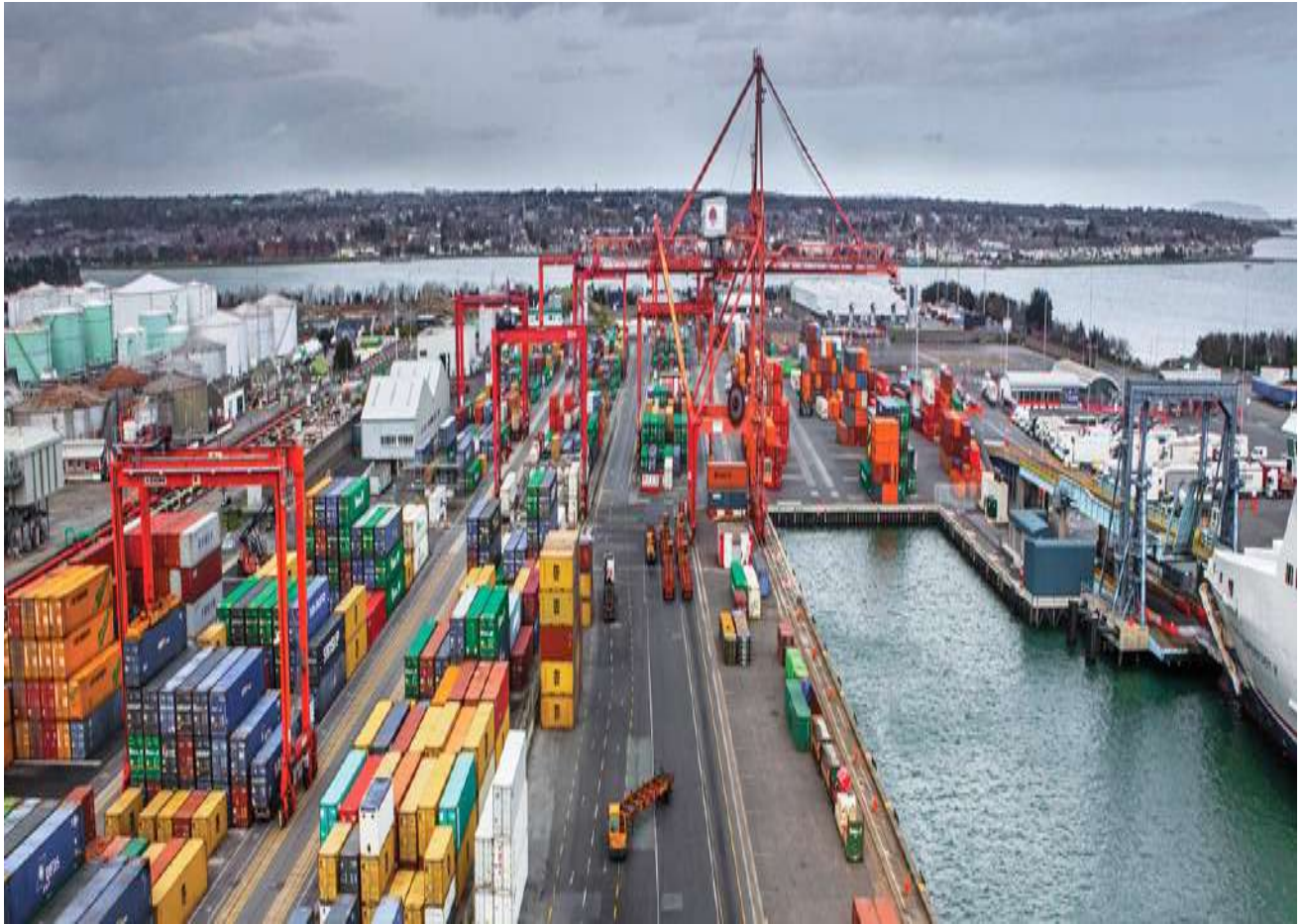
Port of Dublin, Dublin Ferry Terminals (DFT) Berth No.50 North.
