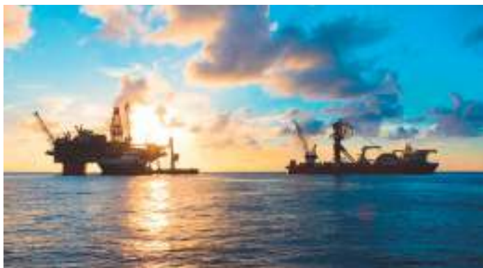
Above: Thunder Horse South Expansion project in the US Gulf of Mexico.
