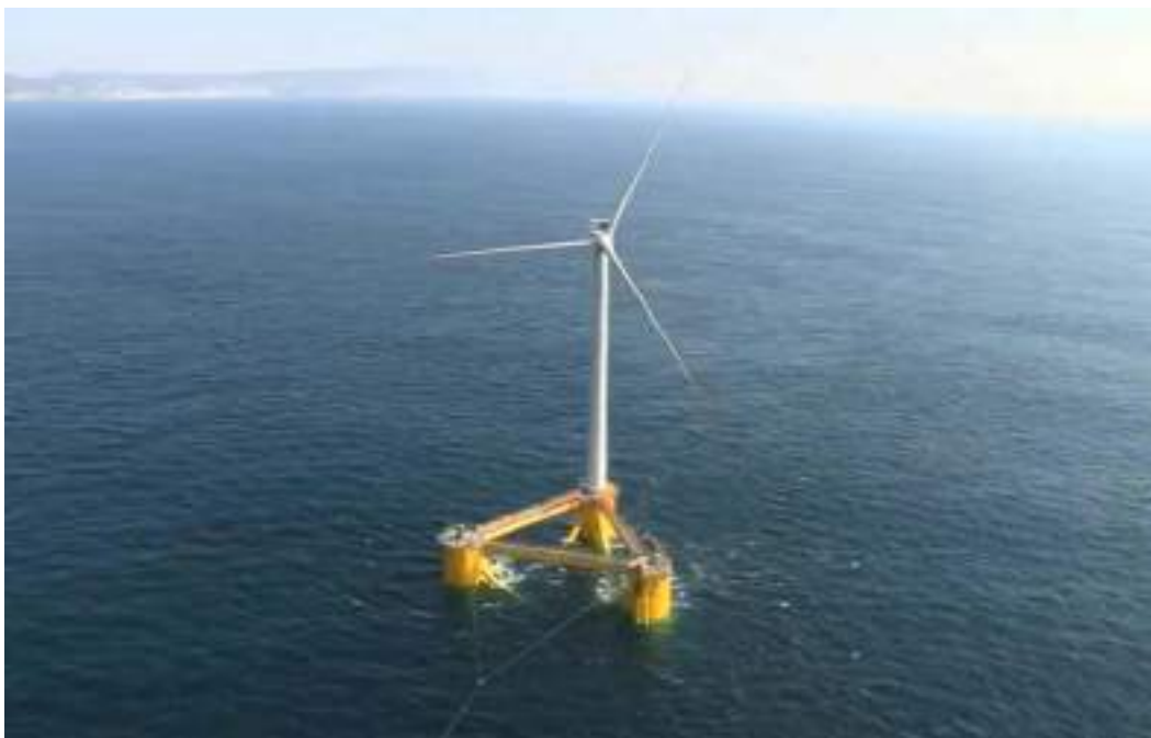
Figure 9 A floating wind turbine
