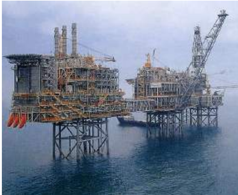
Figure 17 An example of a Production Platform
