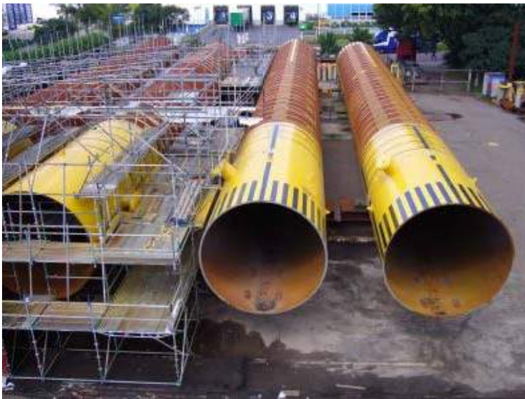
Figure 15 Typical underwater piping
