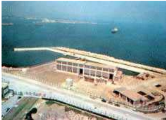
Figure 19 A Seawater Intake / Sewage Outfall
