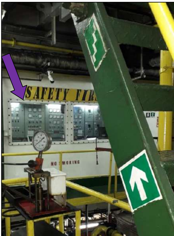
Figure 2: Engine control room window
