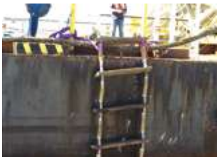
Figure 3 – Ladder supported by strops and not the side ropes
