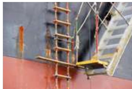
Figure 6 – Ladder not attached to hull
