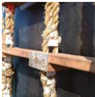
Figure 12 – loose chocks – spreader replaced and not constructed of one piece of wood
