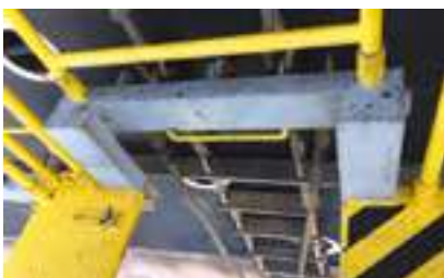
Figure 9 – Pilot has to lean back to gain access to trapdoor
