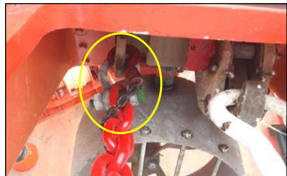
Figure 2: Chain block assembly at the lifeboat's side. The other end of the chain block was attached to the stairs leading to the lifeboat's embarkation platform
