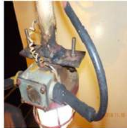
Repaired light foundation at nav. deck
