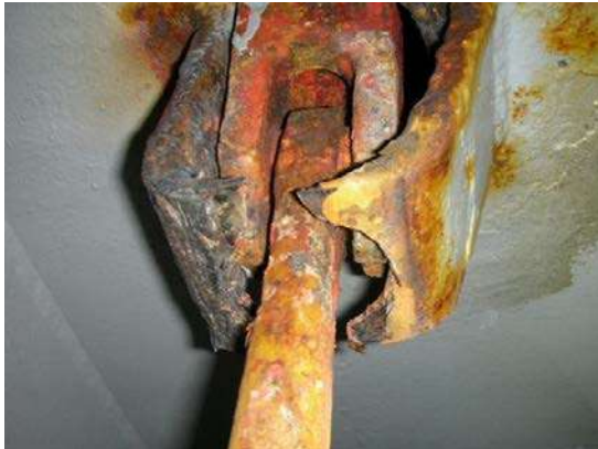
Hatch cover securing device wasted and badly corroded.
