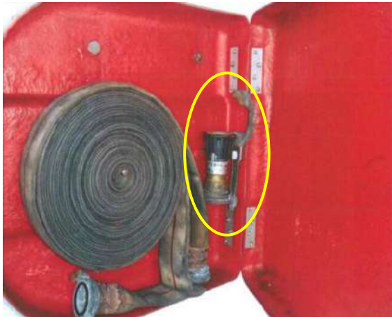
Properly fitted hose nozzle.
