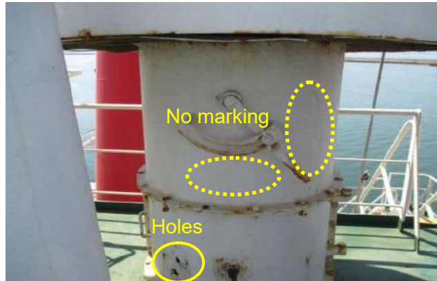
Holes in ventilation trunk and "Open-shut" positions not clearly marked.
