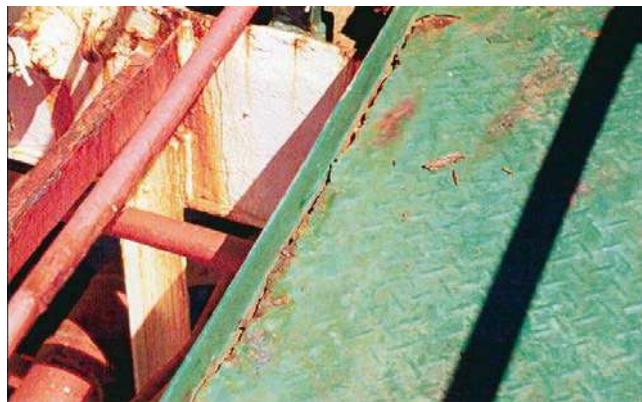
Catwalk cracked.
