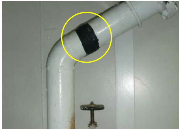
Pipe temporarily repaired with rubber patch.
