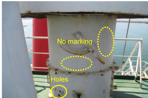
Holes in ventilation trunk and "Open-shut" positions not clearly marked.
