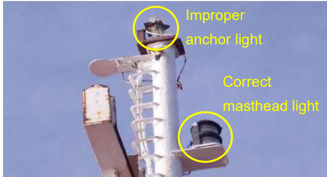
Signal light installed improperly as anchor light. Correct masthead light is to cover a 225 degree arc of the horizon.
