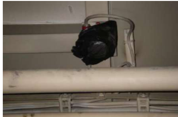
Smoke detector covered by plastic bag.
