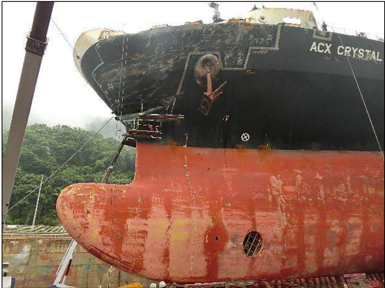
Figure 9. Postaccident damage to the ACX Crystal's bow. (Source: Japan Transport Safety Board)
