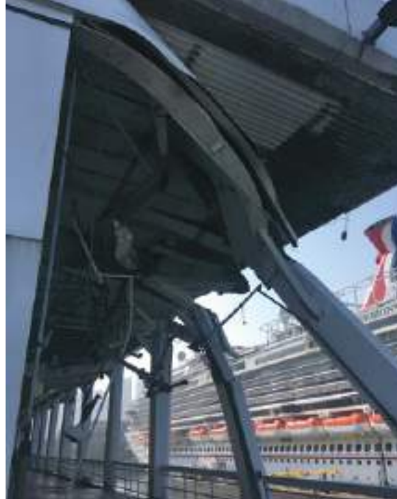
Figure 56. Structural damage to Pier 90's parking garage.
