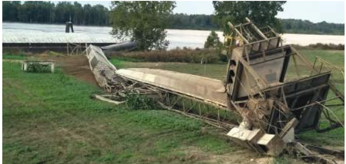
Figure 45. Damaged conveyor as seen from the bank looking toward the river.
