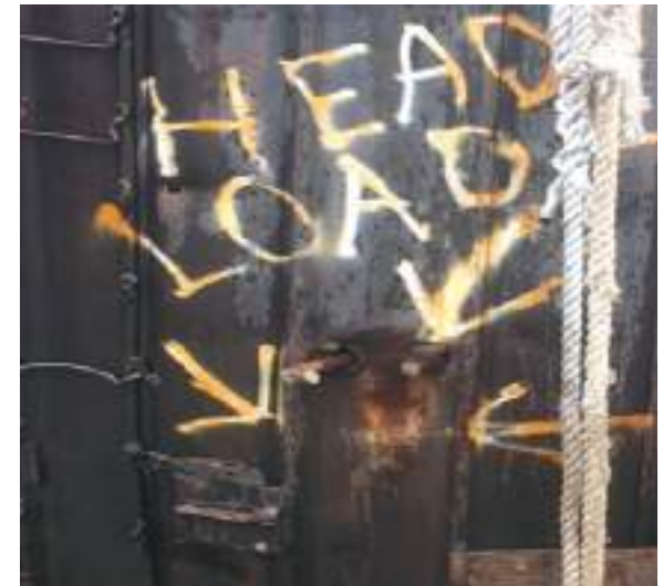
Figure 51. Below, the forward piling at Jacks Run with a broken mooring ring anchor point and missing ring.
