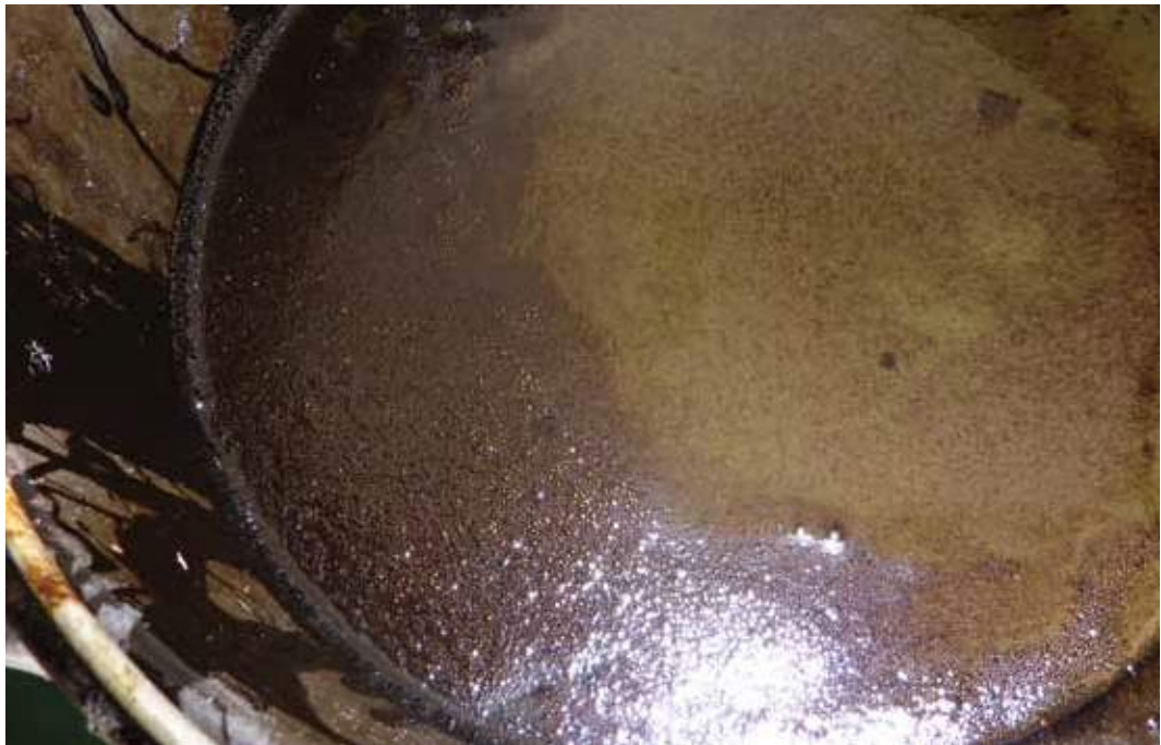
^ Check bunkers for signs of frothing
