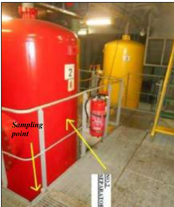
Figure 9: Location of LEL and O 2 sampling point
