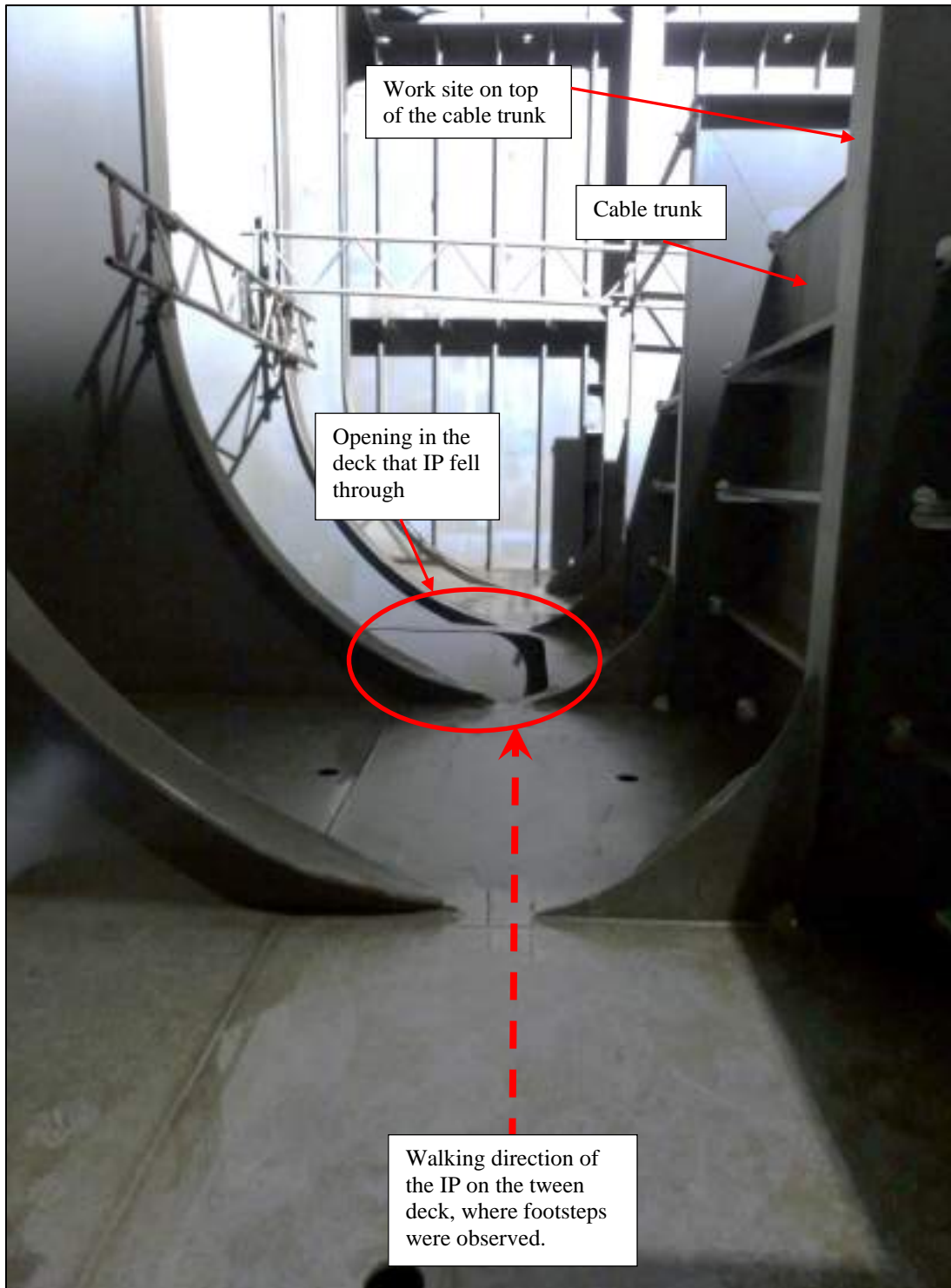
Figure 12: Access ladder passing cable trunk. Lighting conditions are similar to those at the time of the accident
