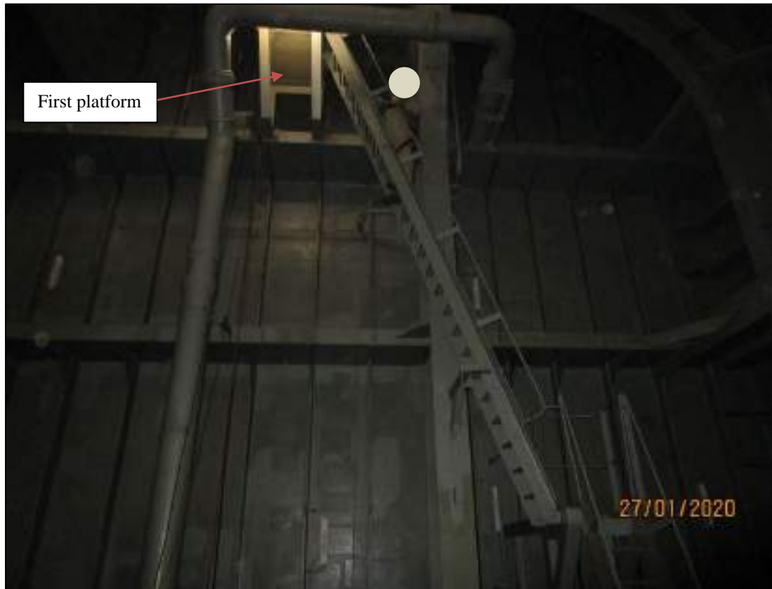
Figure 9: Access ladder inside water WBT no. 1006
