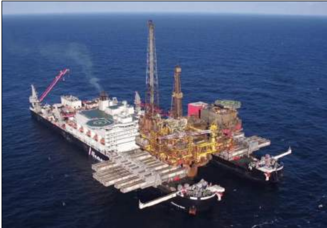
Figure 2: Pioneering Spirit carrying topside
