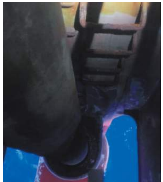
Image 2: Internal ladder housing
