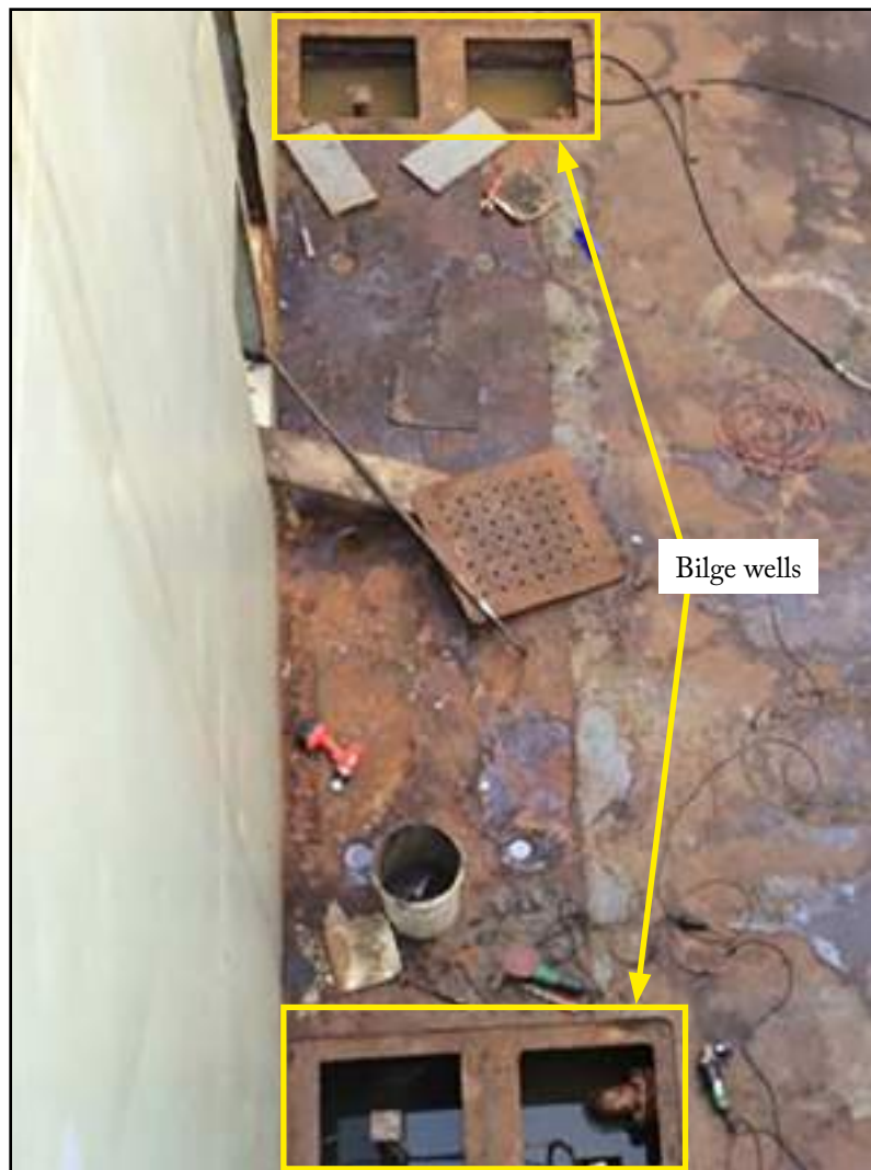
Figure: Cargo hold bilge wells
