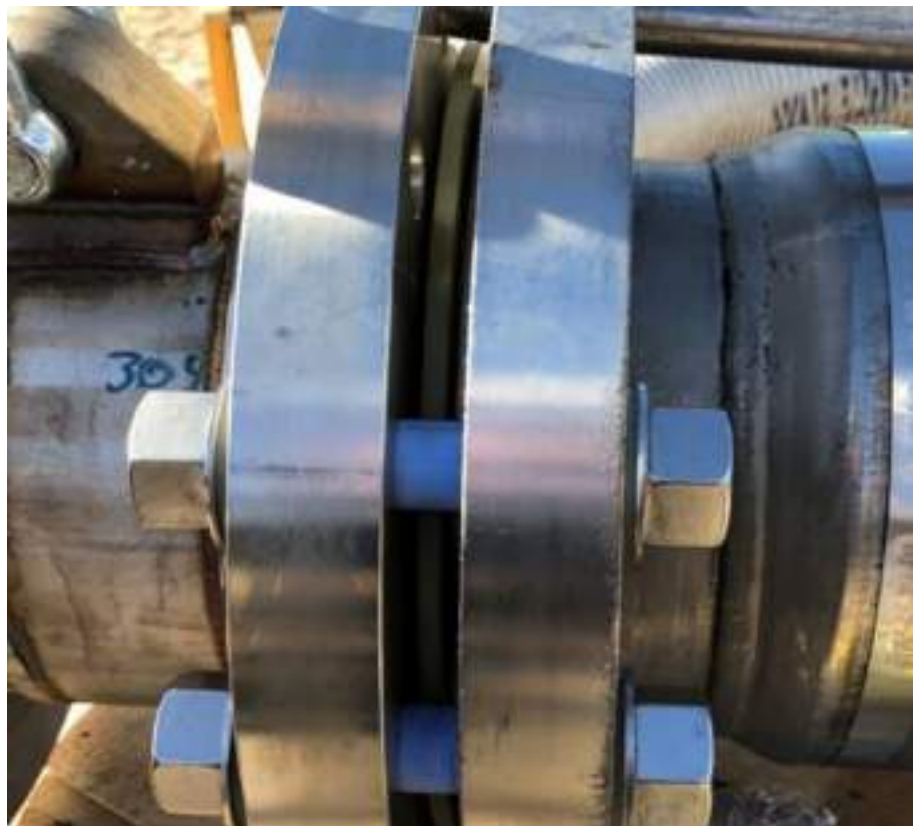
Figure 5.5: Example of a Type 1 Insulator – insulating gasket kit
