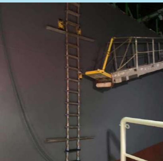
Accommodation ladder's lower platform is not horizontal with waterline.
