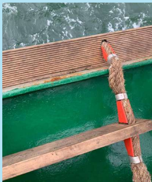
Wear and tear on the pilot ladder rope will occur at a faster rate if no sharp edge protection is in place.
