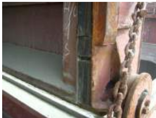
Figure 6: Section replacement of rubber seal
