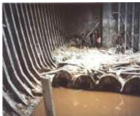
Figure 1: Cargo damage due to water ingress
