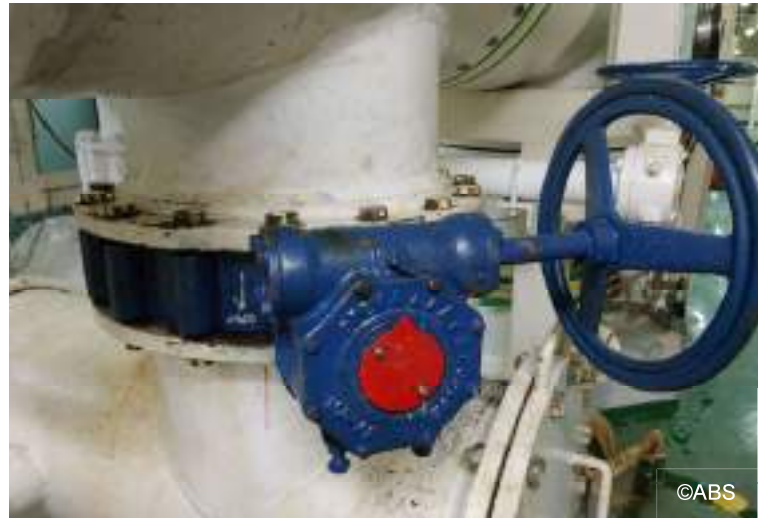
Handwheel for SW valve for central cooling replaced
