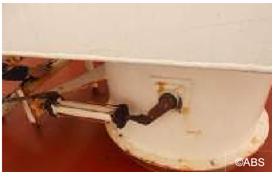
Fire damper linkage repaired
