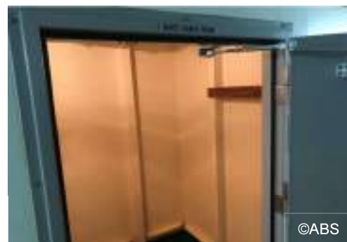
Self-closing fire door after repair
