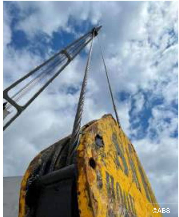
Cargo crane wire renewed – after
