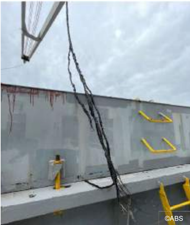
Cargo crane wire parted - before
