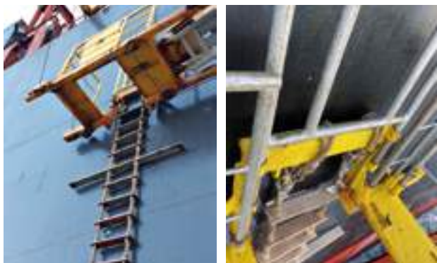
2 examples of non-compliant 'trapdoor' pilot boarding arrangements
