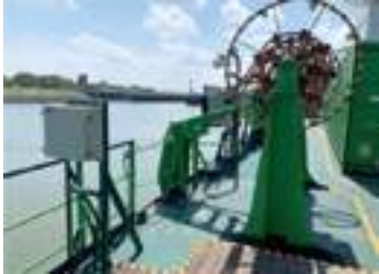
Non-compliant (by design) pilot ladder winch.
