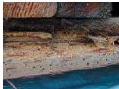
Figure 6.13 Wood frass from boring insect
