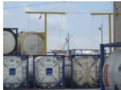
Figure 8.12 Fall arrest stanchions
