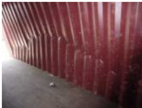
Figure 7.50 Damaged CTU side wall
