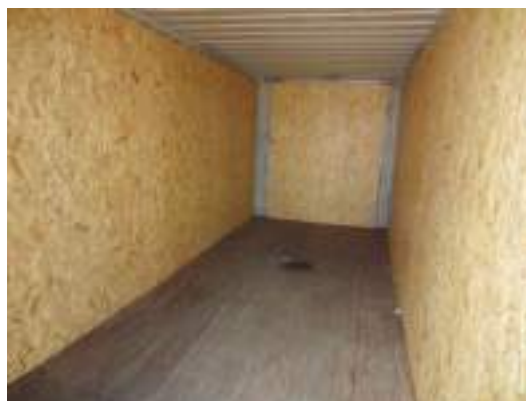
Figure 7.53 Lining a 40-foot container with chipboard panels
