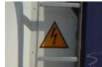
Figure 8.5 Overhead warning sign
