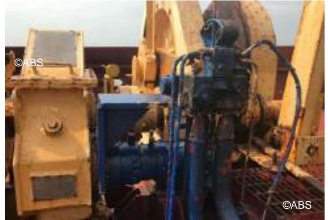
Damaged hydraulic motor for mooring winch replaced
