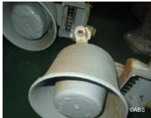
Public address speakers not functioning
