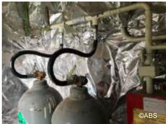
Paint store CO 2 hoses replaced
