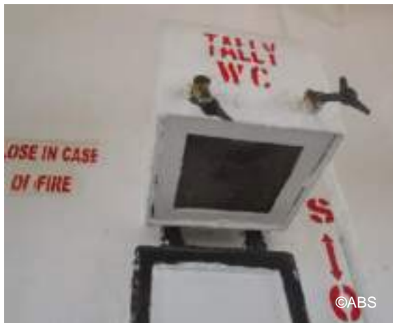
Ventilator dog broken/missing
