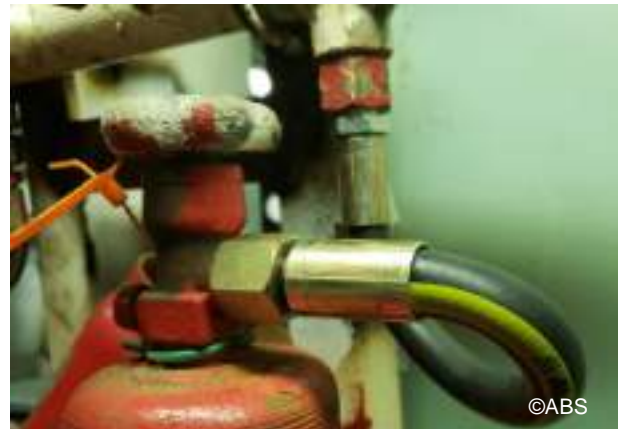
Deteriorated hose for CO 2 system for scavenging air system replaced
