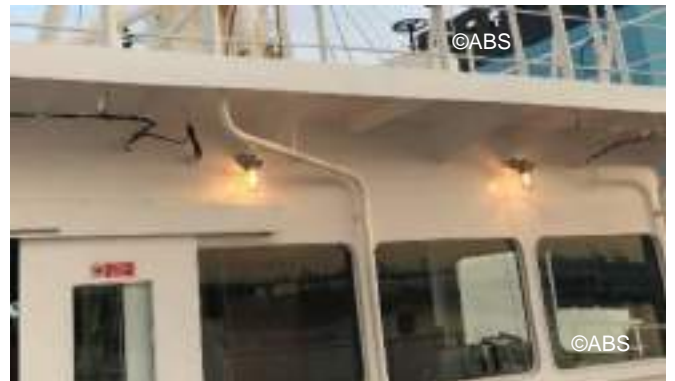
Operational test of emergency lights after repair
