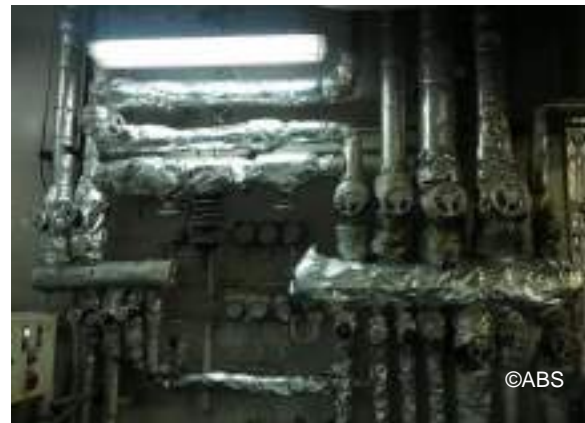
Missing pipe insulation restored
