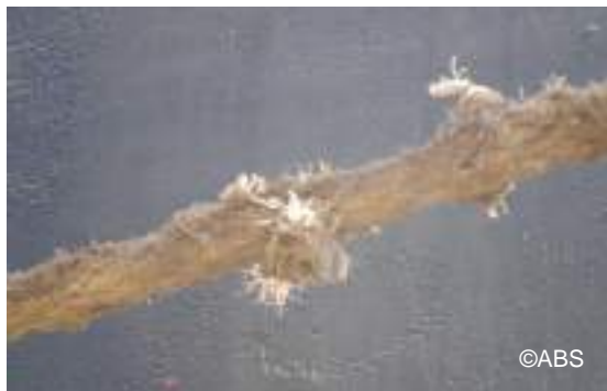
Mooring rope with broken strands
