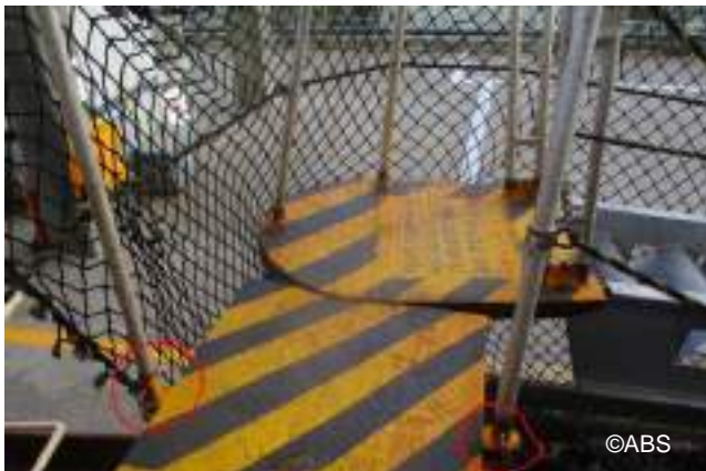
Stanchions secured with locking pins - after
