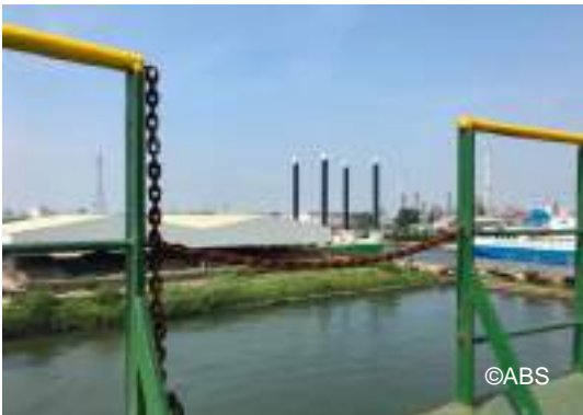
Missing chains for crew protection
