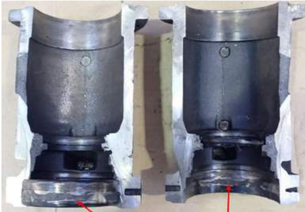
Thermal oil pump #1's bearing housing, split longitudinally. Arrows show the drive end bearing's outer race fused to the housing (left) and heat affected longitudinal band (right).
