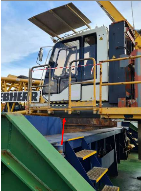
Figure 6: Access to the crane from starboard side
