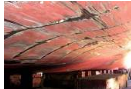
▲ Bottom damages as a consequence of machinery failures 1
