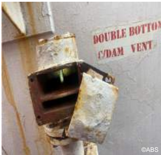
Ballast tank vent head disk missing
