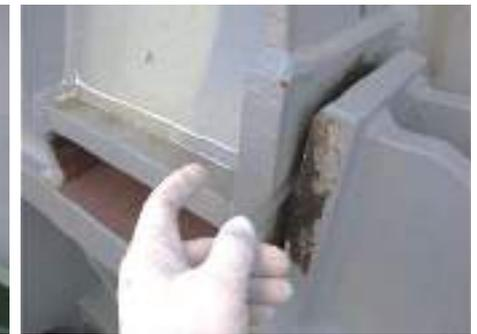
Photograph 14 Measuring clearance of locator with tapered feeler gauge.
