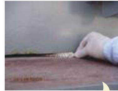
Photograph 11 Checking skirt clearance with feeler gauge
