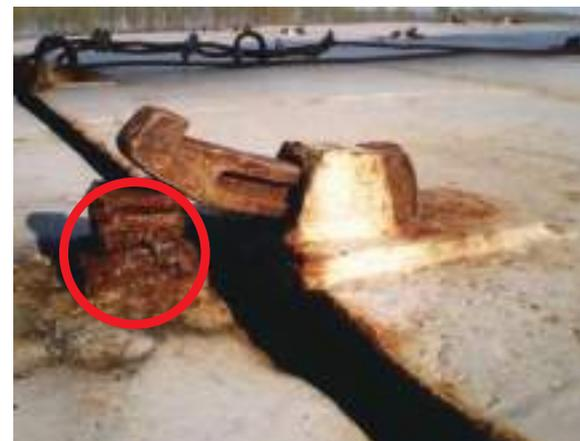
Photograph 17 “Banana shaped” cross wedge with striker plate built up
