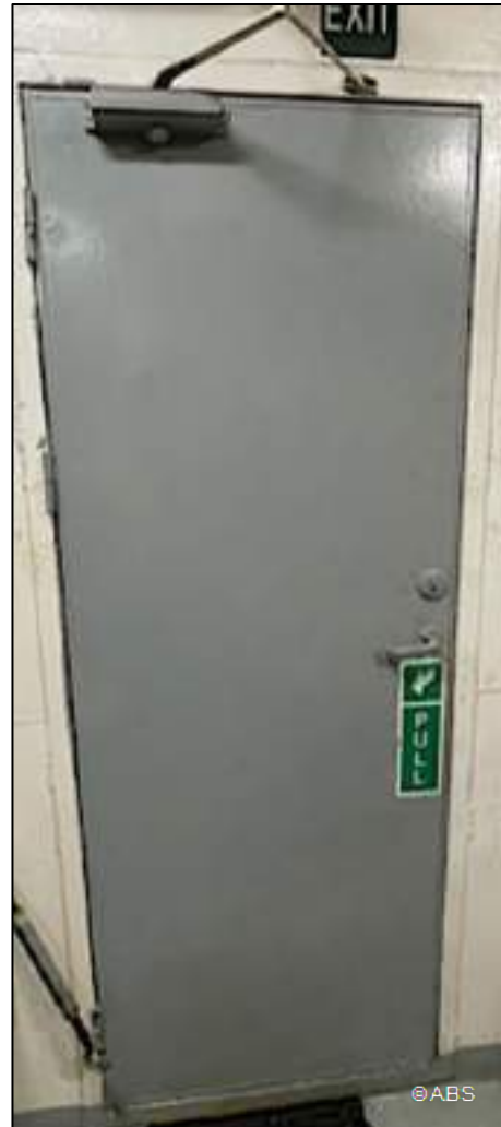
Fire door in poop deck does not close properly
