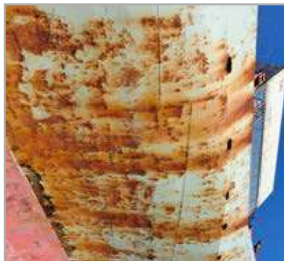
Hull corroded [corroded]
