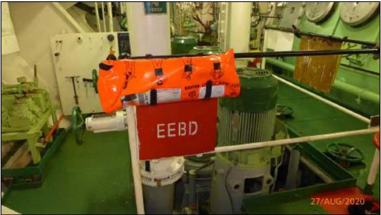
Figure 24: EEBD location at the entrance to the bottom deck emergency escape
