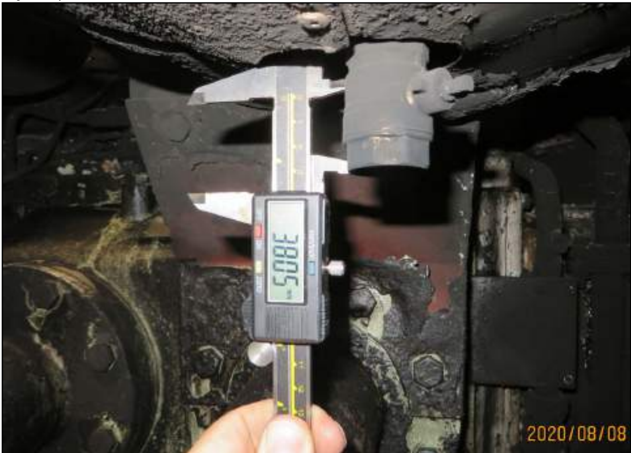
Figure 22: AE2 exposed turbocharger water washing drain connection
