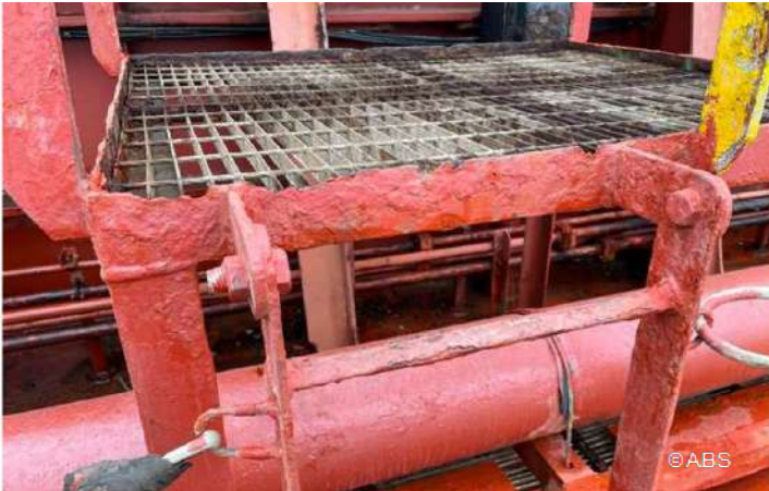
Standing platform excessively wasted
