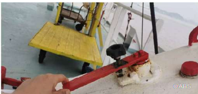
Rescue boat winch speed engaging lever inoperable
