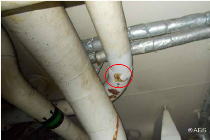
Ballast pipe repaired with patch
