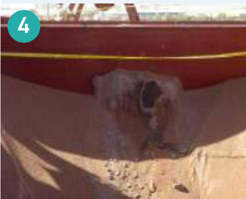
Figure 4: Column/area of wet damaged cargo positioned beneath the hatch cover joint.
