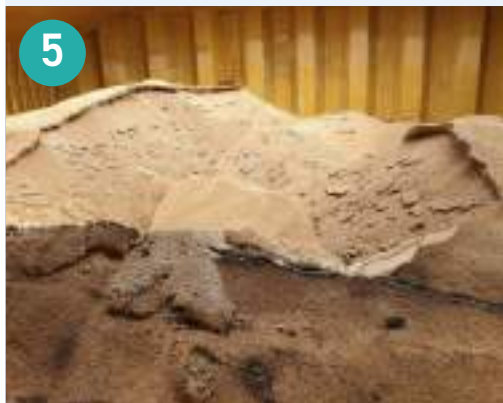
Figure 5: Partially discharged stow of soya beans with characteristic mouldy crust on the surface due to self-heating within the pile. The dark black discolouration is a drip line due to condensation dripping from the interior steelwork.
