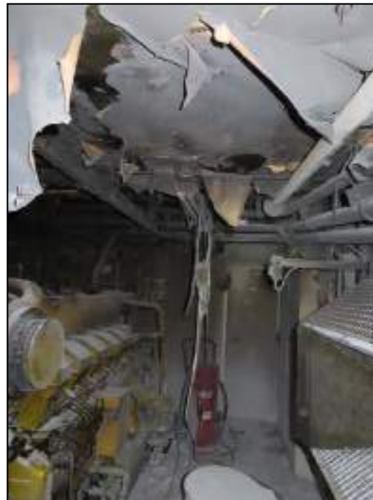
Finnmaster's fire-damaged compartment
