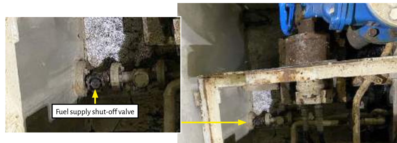
Figure: Fuel supply shut-off valve
