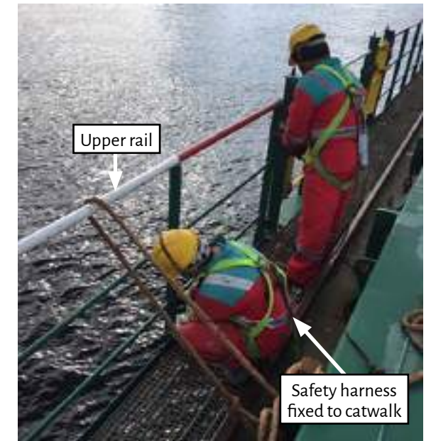
Figure 1: Bolts being removed from a section of upper rail
