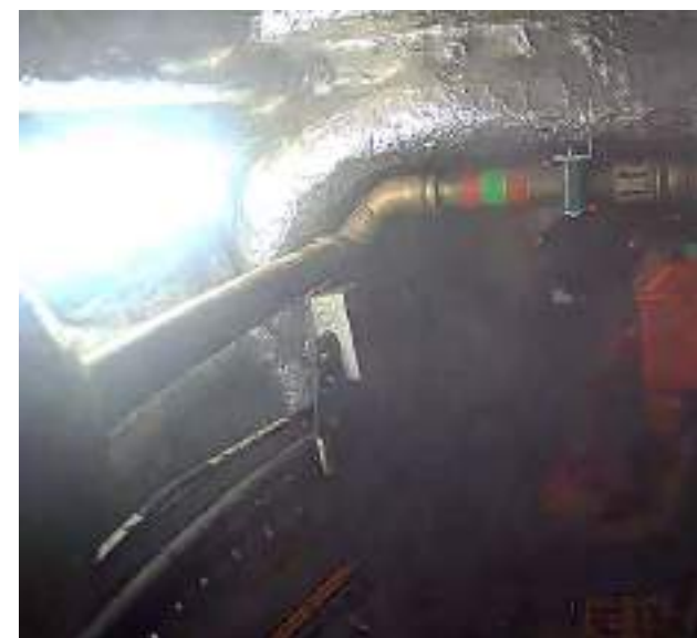
Figure 1: CCTV still showing smoke in engine space
