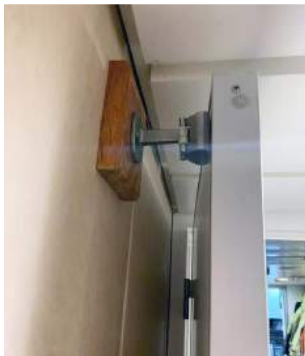
Figure 1: The hold-open mechanism on the door
