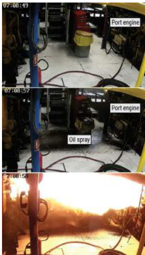
Figure 77. Screenshots from the Capt. Kirby Dupuis engine room video camera (looking aft).
