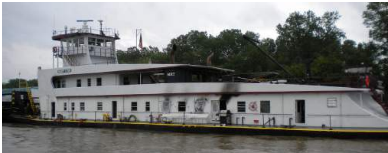
Figure 83. Mary Lynn 's port side, postcasualty, with some of the plastic window coverings remaining over the engine room windows. SOURCE: COAST GUARD
