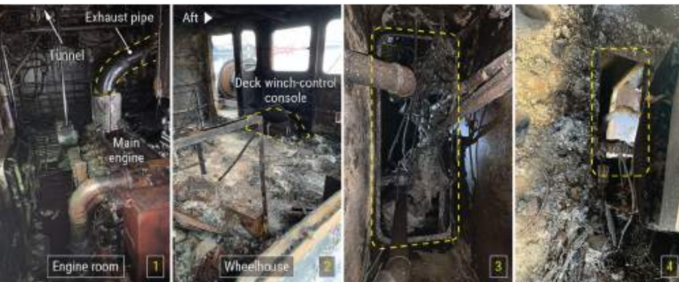
Figure 94. Left to right: Post-fire damage of (1) the engine room, where the crew removed the lagging from the exhaust pipe, as indicated by the dashed line; and (2) the wheelhouse, where the captain observed black smoke emanating from under the deck winch-control console. Damaged pipe/hose tunnel, as identified by dashed rectangles, looking up from the engine room (3), and down onto the deck winch-control console location (4).
