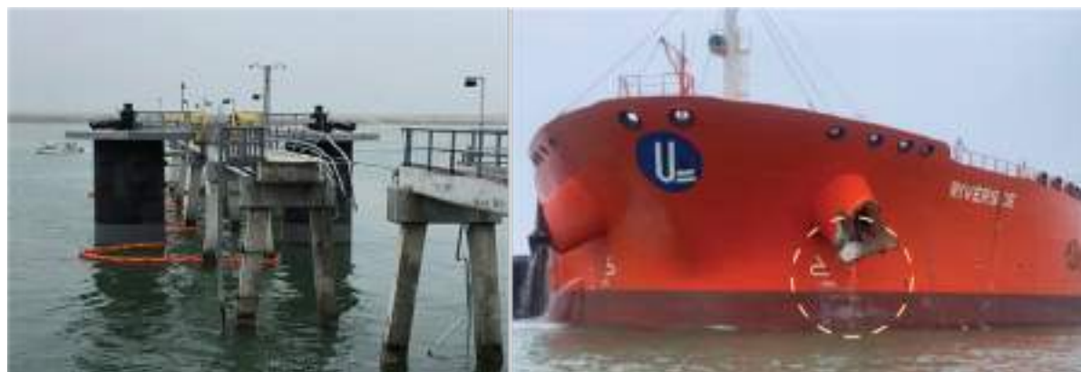
Figure 58. Damage to the no. 4 Moda dock catwalk (left) and the Riverside (right, circled). SOURCE: COAST GUARD
