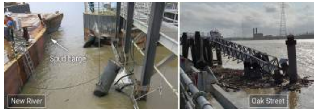
Figure 118. Left to right: Damage to the river intake fender systems: arrow shows damage to the spud barge at New River; damaged catwalk and dolphin piles at Oak Street.
