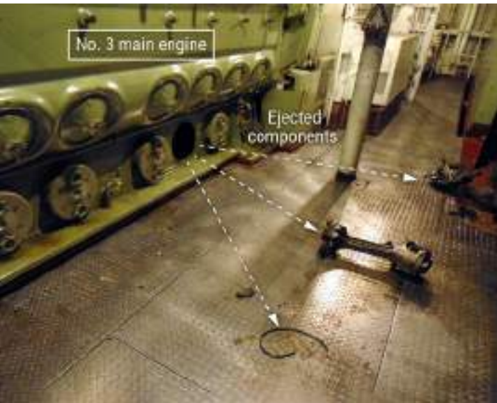
Figure 138. Ejected components from the no. 3 main engine. BACKGROUND SOURCE: COAST GUARD
