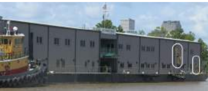
Figure 47. Office barge with detached mooring apparatus and structural penetrations (outlined in white).
