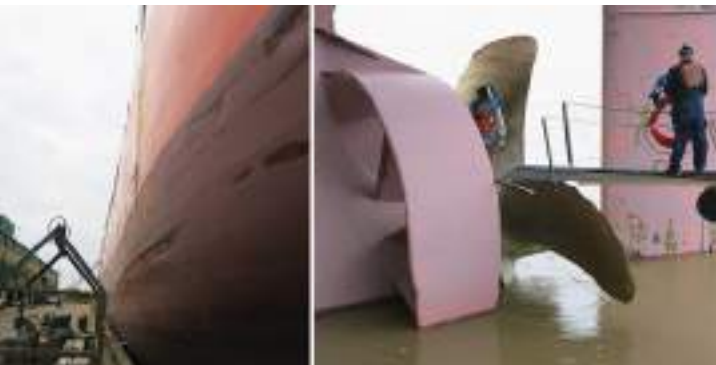
Figure 114. Below, left to right: Postcasualty damage to the Bow Tribute's portside aft hull and propeller.
