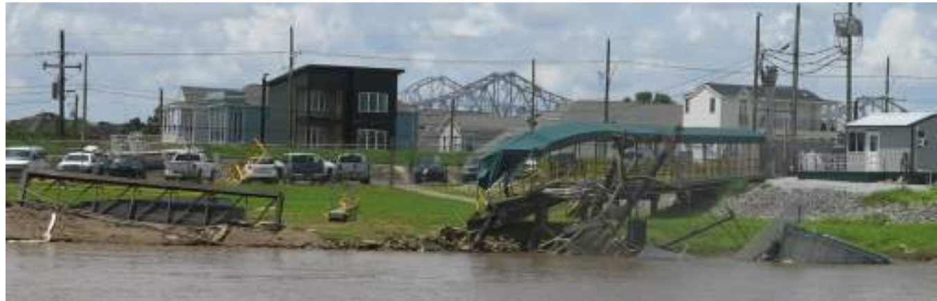
Figure 45. Postcasualty damage to office barge moorings, catwalks, and gangways.
