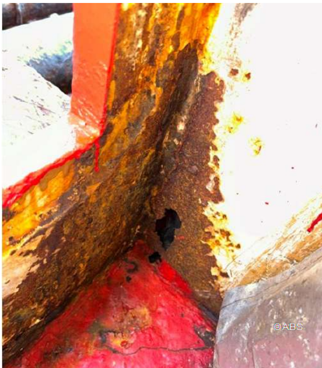
Emergency escape to main deck from engine room, structure wasted with holes
