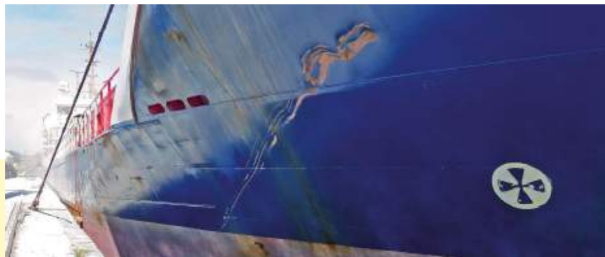
Figure 3: The area of plate damage
