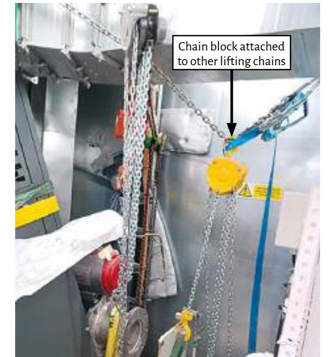
Figure 3: The lifting arrangements
