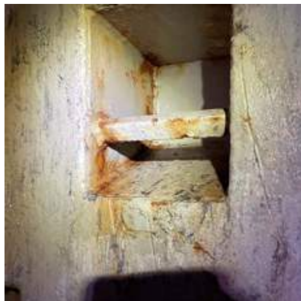
Figure 1: A recessed foothold
