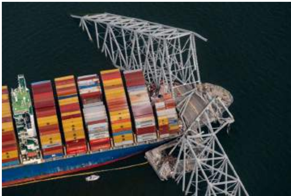
Wreck of the DALI intertwined with the bridge in the Fort McHenry Channel.
