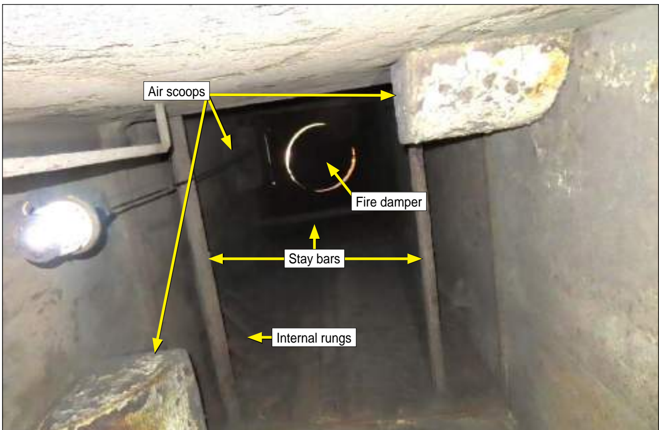
Figure 5: Starboard ventilation trunk internal structure, looking up from the access cover
