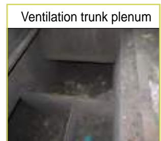
Figure 3: Starboard engine room ventilation duct arrangement
