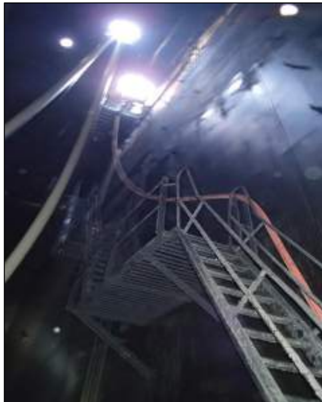
Figure 11: Port side slop tank after the accident
