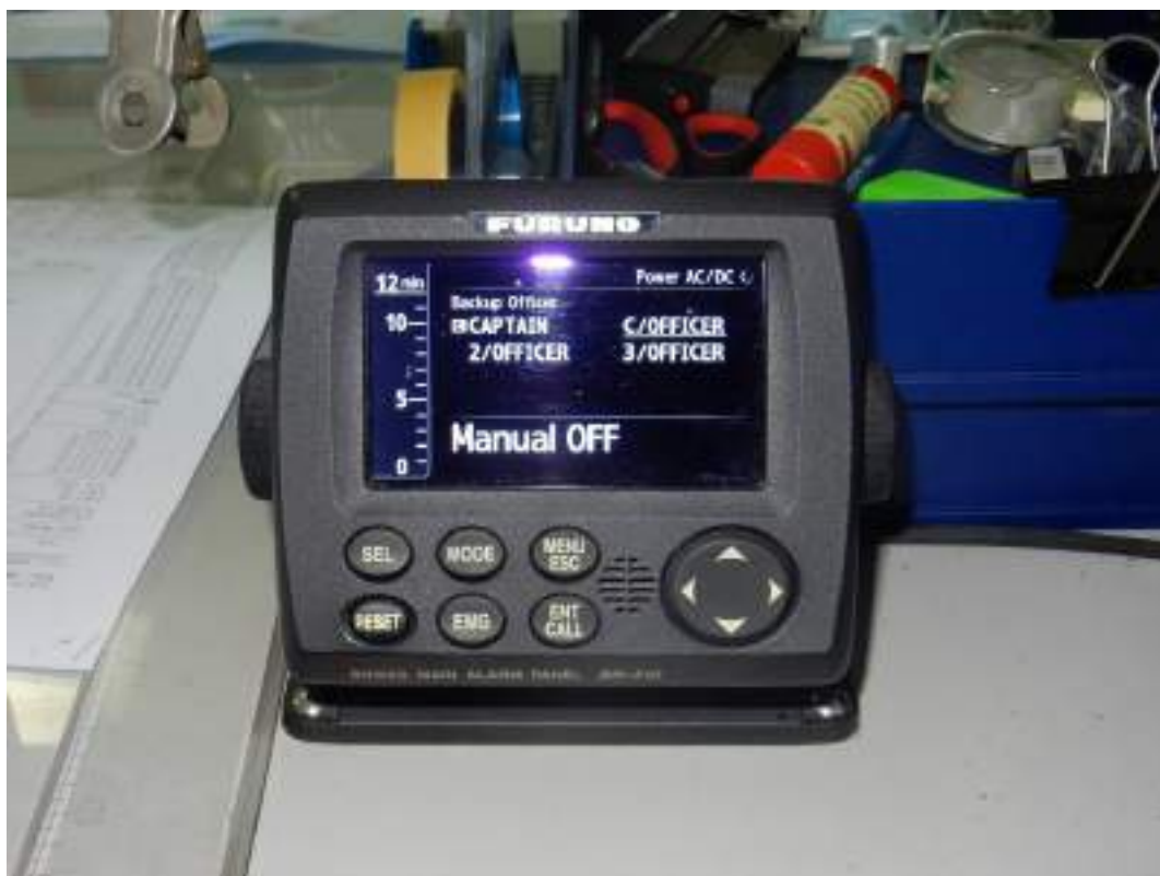
Photo 3. The vessel's BNWAS (Bridge Navigation Watch Alarm System). Photo: SHK.
