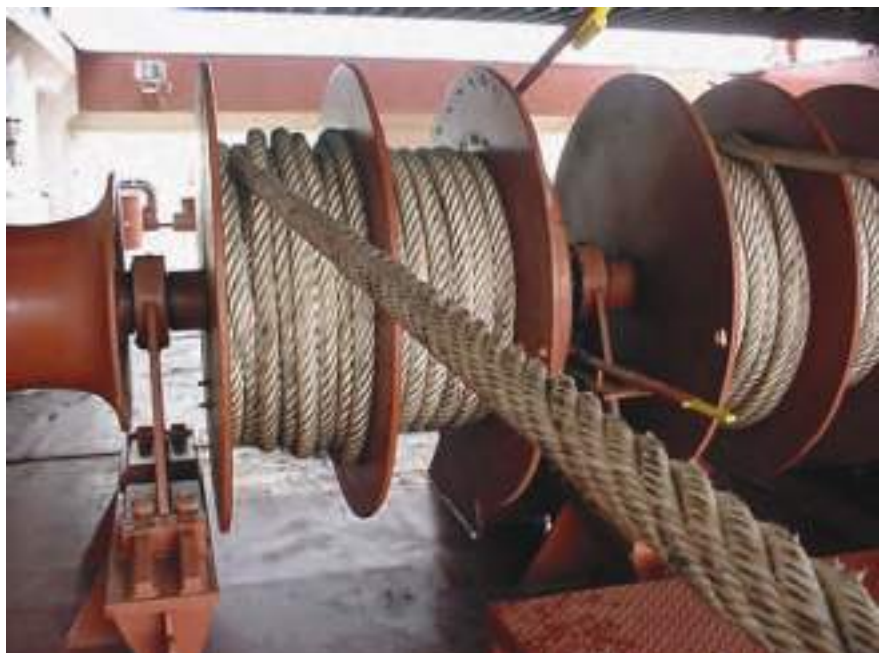
Incorrectly set up split drum with buried mooring line
